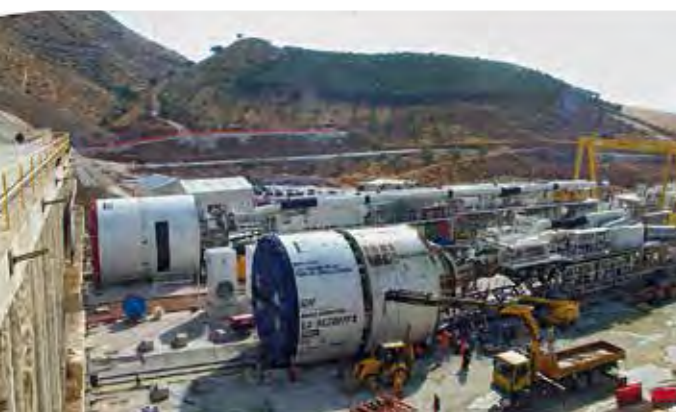
Train testing in the Guadarrama tunnel in June 2007 (above). Below, excavation of the Abdalajís tunnels (Córdoba-Málaga HSL) with TBMs (2006).
