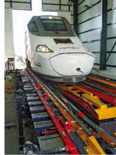
From left to right, variable gauge changeover installation; Ineco has designed a large number of these and is responsible for the maintenance of 16 throughout Spain. Víctor Duarte, a civil engineer, in 2003 on the works of the Córdoba-Málaga line.
