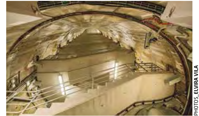
High-speed tunnel between Atocha and Chamartín, Madrid, for which Ineco managed the works and provided assistance in soundings and geotechnics. Above: Emergency shaft. Centre: Álvaro García Tapia and Juan Martínez working on signalling in 2017. Below: TBM receiving shaft in Atocha, 2011.
