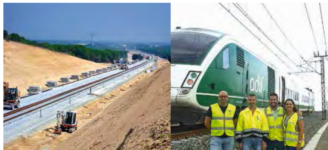
Above, the Madrid-Lleida line: installation of overhead lines (left) and the arrival of the first high-speed transformer at Peñalba station in 2001 (right). Below, works on the Madrid-Valladolid line in 2007 (left) and Ineco's Traffic team in 2017 (right).
