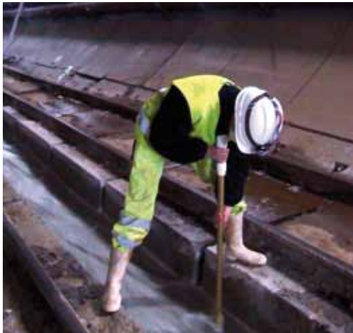
RIGHT: An assessment inside one of the Pajares Tunnels to monitor the flows drained from each aquifer system crossed.
