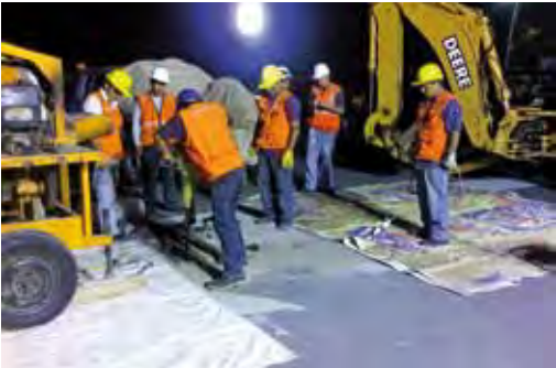
THE INECO-CPS TEAM From left to right, Anibal Ormeño and Juan Medina, both from CPS, along with Ángel Toro, from Ineco, during a nighttime pavement inspection. To the right, drilling work on the pavement in order to characterise the pavement package and foundation.
