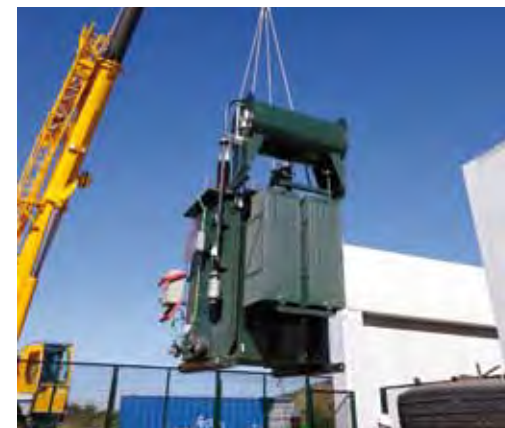
Transportation of equipment to an auto-transformation centre on the Ourense-Santiago section of rail.
