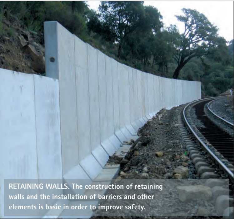
TRACK ASSEMBLY. The existing fill was replaced with sandy ballast and new PR-01 and AM-05 multi-purpose sleepers were installed, as were 60 E1 and UIC-54 rails.
