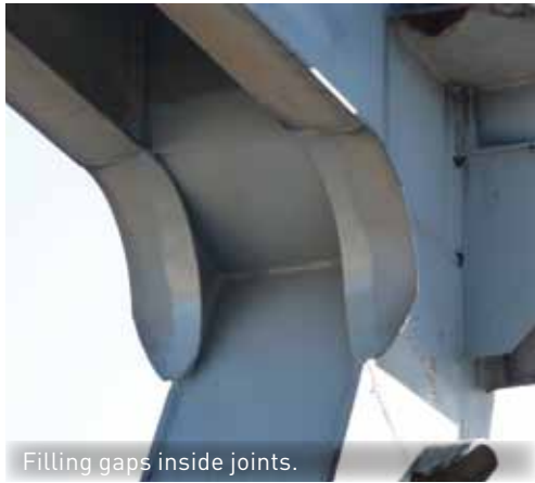
Filling gaps inside joints.
