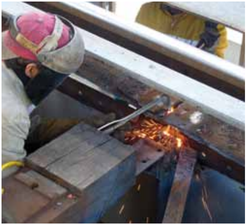
REMODELLING THE DECK This image and the two images on the right show workers replacing and reinforcing the top wings of the rail bearers.
