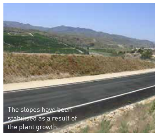
The degree to which the planted vegetation has taken root is very high, despite the harsh edaphoclimatic conditions of the land.
