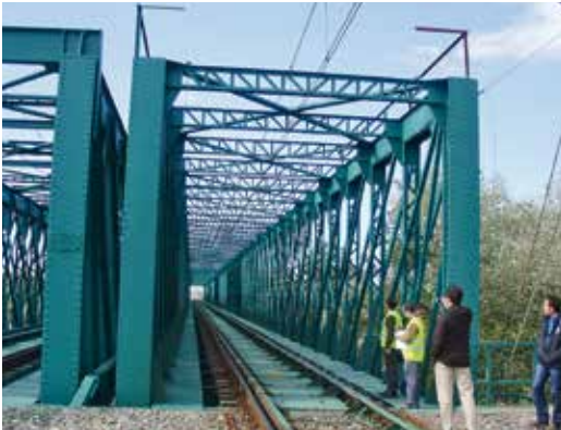
ALCÁZAR DE SAN JUAN-SEVILLE LINE K. P. 523 + 467 / Track 1 The bridge has five sections with a total length of 254.400 m. It has two main continuous beams, with a theoretical span of 50.760 m in each section; with a Linville truss of 18 modules per section, and a 6.28 m abutment edge.
