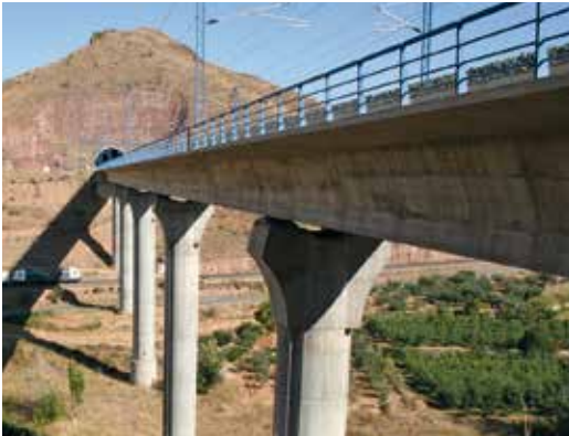
HIGH SPEED LINE MADRID-BARCELONA K. P. 239 + 429 / Section Calatayud – Ricla Continuous prestressed concrete deck with box section and concrete piles. Total length is 250 m, in six spans, two of 35 m and the four central ones of 45 m. The 96 points with regular technology instruments were supplemented with an additional network of 16 sensors and FBG equipment.
