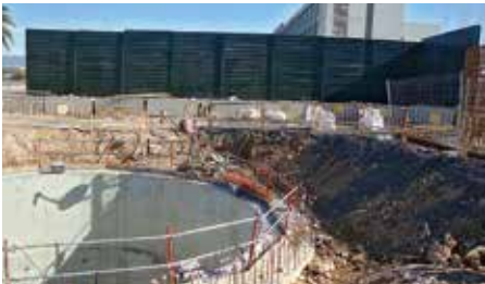
Temporary acoustic screen installed to protect the hotel, located next to emergency exit No. 2.
