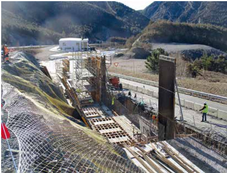
The photos above show the response to one of the biggest challenges of stabilising the embankments using retaining walls and metal netting to prevent landslides and falling debris.
