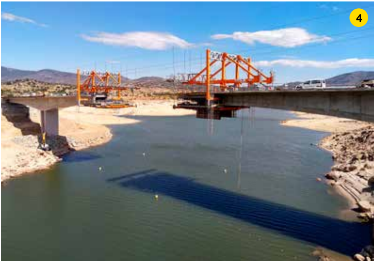
4. The new bridge was constructed using the incremental launching method for the central section and falsework for the ends, while the old bridge (5) was constructed using rigid movable falsework.
