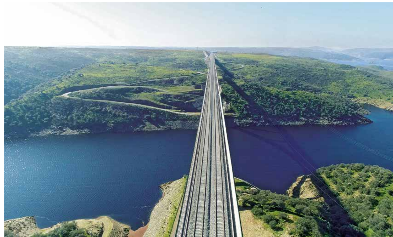
The imposing Almonte viaduct (996 m long) is part of the new Madrid-Extremadura high-speed line between Plasencia and Cáceres, passing over the Alcántara reservoir with a concrete arch spanning 384 m, making it the world record holder for railway spans.
