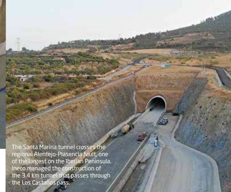
The Santa Marina tunnel was waterproofed using a non-conventional system in order to provide completely watertightness.
