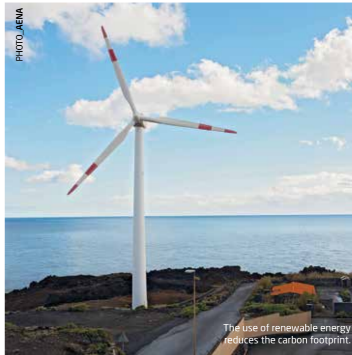
Aena's Photovoltaic Plan will prevent the emission of 167,000 t of CO 2 each year.
