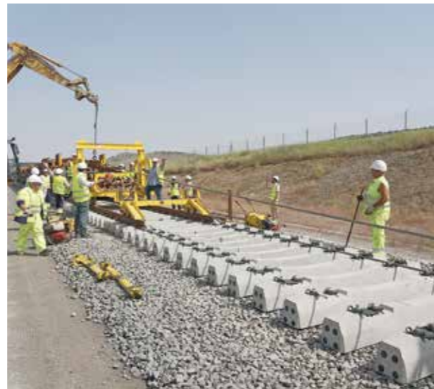
In addition to the rail supplied by rail trains in 270-metre bars, rail in 108-metre bars was supplied on conventional platforms consisting of two sextets, which required the development of a new unloading procedure to optimise work performance.
