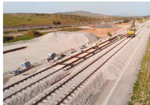
Track assembly work on the section between Plasencia and Cáceres in October 2019.
