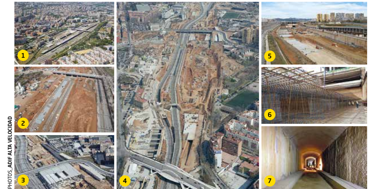
1. Former freight terminal of La Sagrera (2007). 2. Construction of the provisional alignment (2008). 3. Beginning of construction of the logistics area (2013). 4. Beginning of the excavation between screens (2012). 5. Beginning of construction of the floor slab (2018). 6. Close up of the assembly of the floor slab (2018). 7. Completed sewer section of the Rambla Prim (2018).
