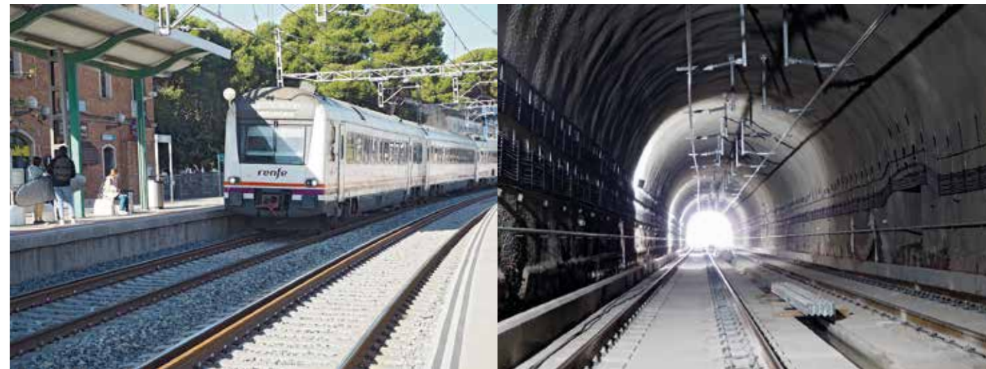
PROGRESS ON THE CONNECTION WITH FRANCE AT VILA-SECA AND THE MARTORELL TUNNEL The works to adapt the Martorell tunnel to standard gauge and the installation of a third track between Martorell and the Vila-seca junction are essential for freight trains to be able to run on standard gauge between Tarragona and Barcelona. The completion of these works will link the road to the area's factories, such as the SEAT factory.
